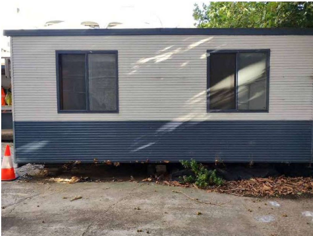
Photo 2: Demountable being used as site office - located in the north east portion of the site
