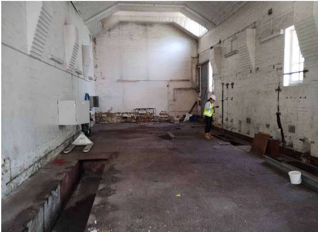
Photo 1: Inside the former electrical substation - person
