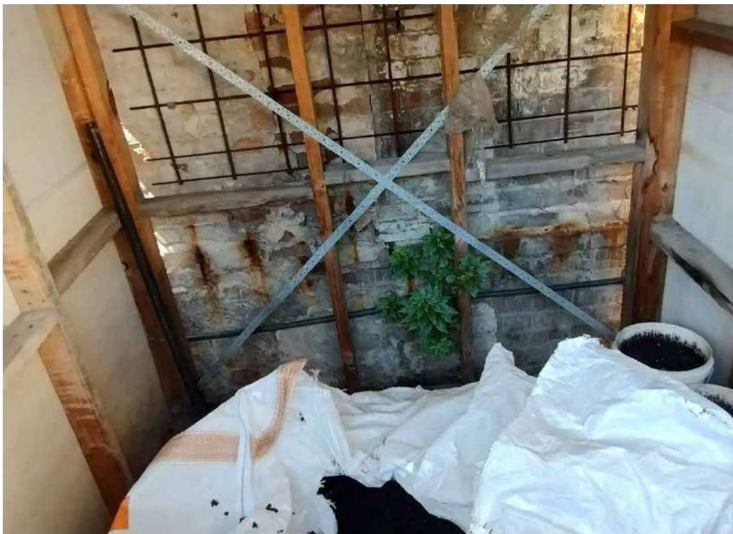
Photo 14: Inside asphalt storage shed in south-west of site
